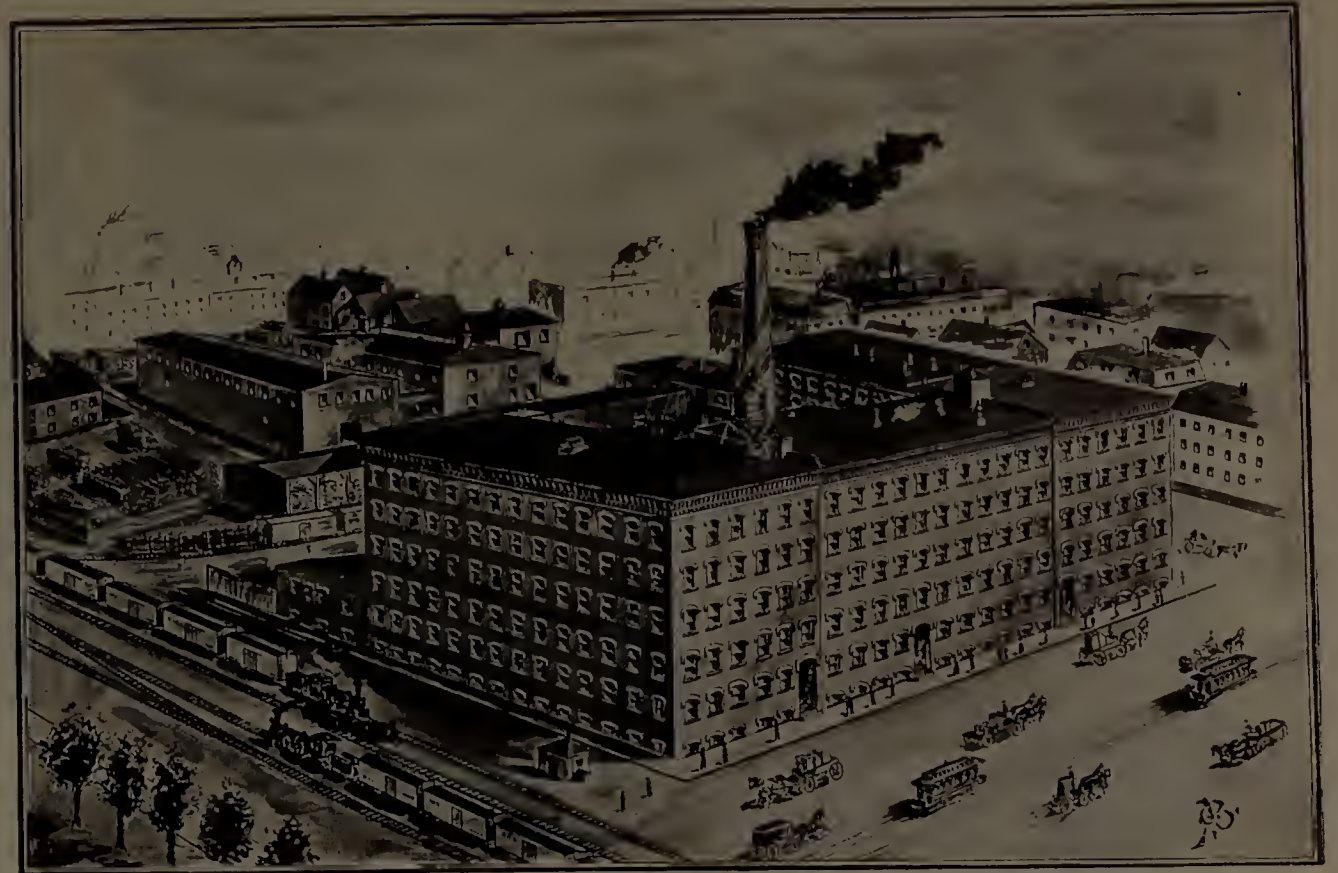
FACTORY OF THE MASON & HAMLIN COMPANY, Cambridgeport. Salesrooms, 146 Boylston Street, Boston.
